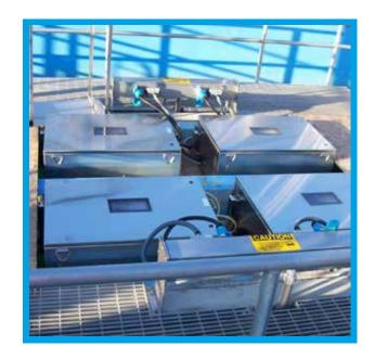
The VCS-40-A150 is our biologically validated vertical amalgam based offering exceeding 1.0 MGD and is designed to treat a 30" water level.
