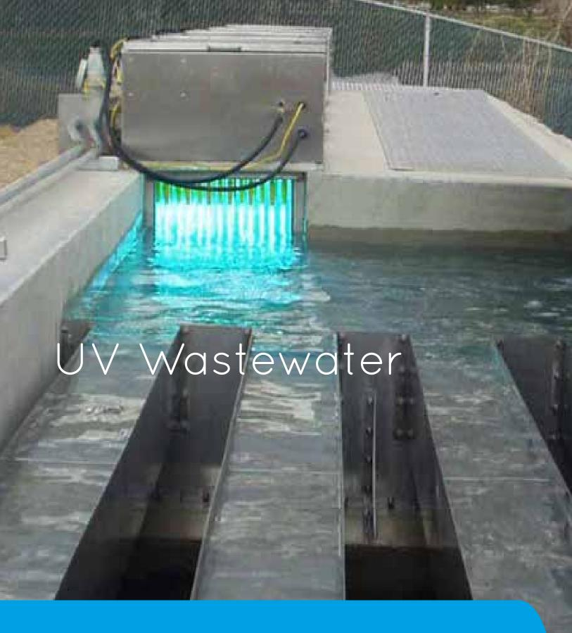
Vertical Open Channel Ultraviolet Disinfection
