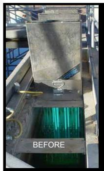
2003. Existing vertical plant using standard 65 watt lamps. Upgraded to high output 155 watt lamps. Allowed the plant to add automatic cleaning and add ability to treat larger flow rates.
