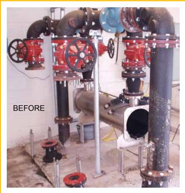
2007 Exising chambered system using low pressure lamps. Upgraded to high output lamps. Allowed the plant to add automatic cleaning and add ability to treat larger flow rates.
