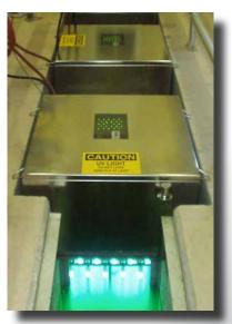
2003. Vertical plant using 65 watt lamps upgraded to amalgam lamps. Allowed the plant to meet more stringent discharge permit.
