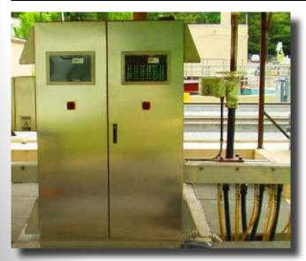
2003. Exising horizontal plant using standard 65 watt lamps. Upgraded to high output lamps. Allowed the plant to add automatic cleaning and ability to treat larger flow rates.
