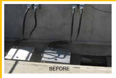
2012. Exising vertical plant using standard 30" - 40 watt 65 lamps. Upgraded to high output lamps. Allowed the plant to add automatic cleaning and add ability to treat larger flow rates.
